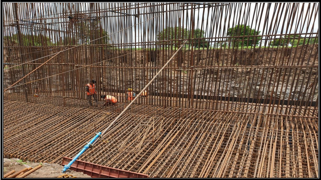
VISIT TO UNDER CONSTRUCTION OF BRIDGE SITE AT WADEGAON, SANGOLA.
